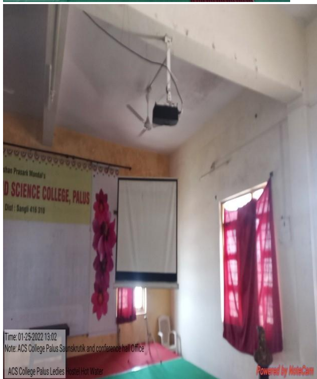
Photo of ICT Room G-4
